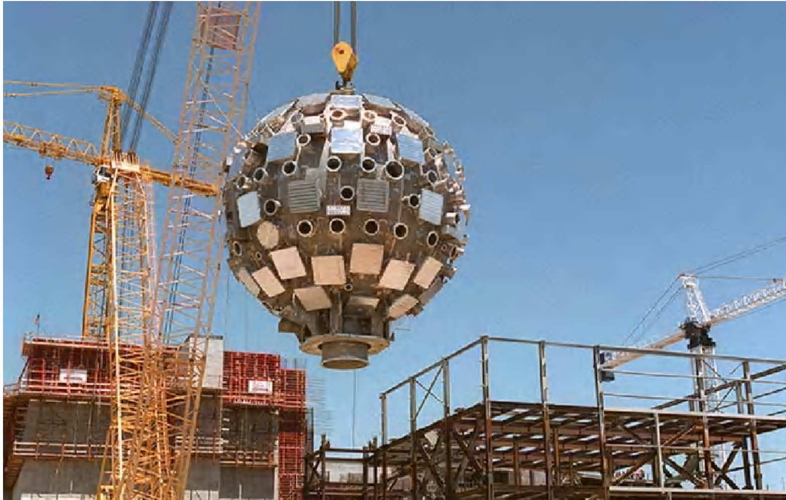
The 10-meter-diameter target chamber, installed in June 1999, weighs 287,000 pounds. The spherical vacuum vessel was assembled from 18 four-inch-thick aluminum sections fabricated by Pitt-Des Moines, Inc., of Pittsburgh, Pennsylvania, and was installed with one of the largest cranes in the world.
